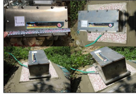
Fig. 9 Photo of on-site installation of geoaoustic instrument
