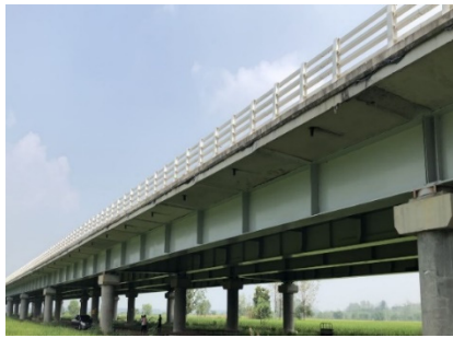
Fig. 10 Photographs of the studied bridge
