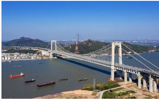
Fig. 1 Wufengshan Yangtze River Bridge
