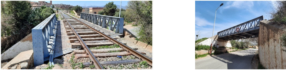
Fig. 1 General view of the bridge of Ouled Mimoun (Tlemcen - Algeria)
