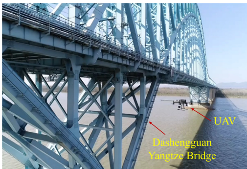
(a) UAV inspection
