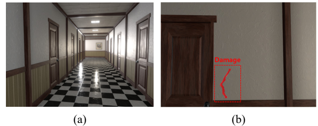
Fig. 2 Examples of captured images: (a) the location looking at an open space; (b) the location closing up the damage
