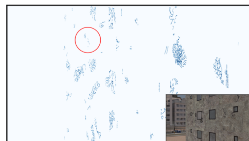
a) Original size crack mask and image
