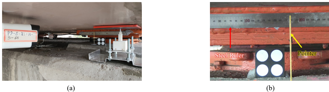
Fig. 14 Installation of analogue displacement meter setup: (a) wide view; and (b) close view
