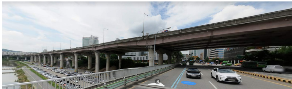
Fig. 10 Overview of Tancheon overpass
