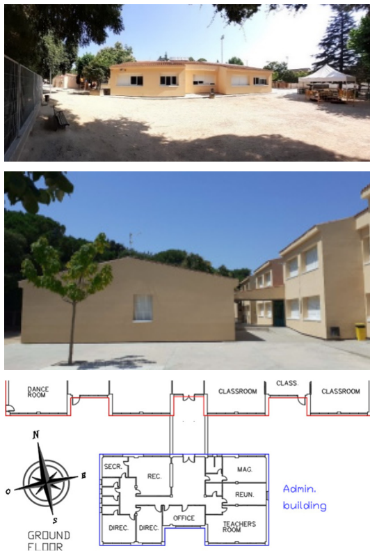
Fig. 2 The administrative building where the tests were carried out
