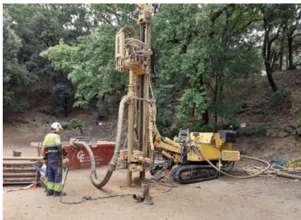
Fig. 7 Drilling site and operation
