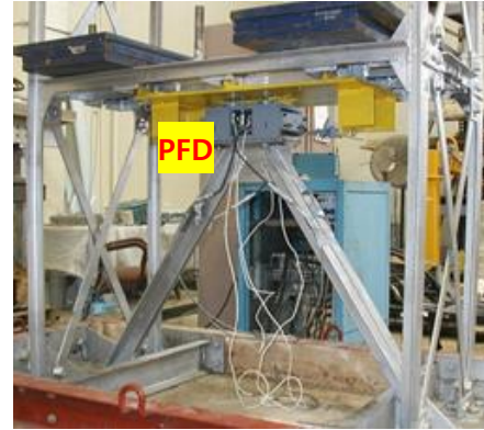
(b) The installation of PFD
