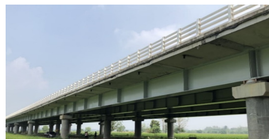
Fig. 4 The Shouchun Huaihe river bridge
