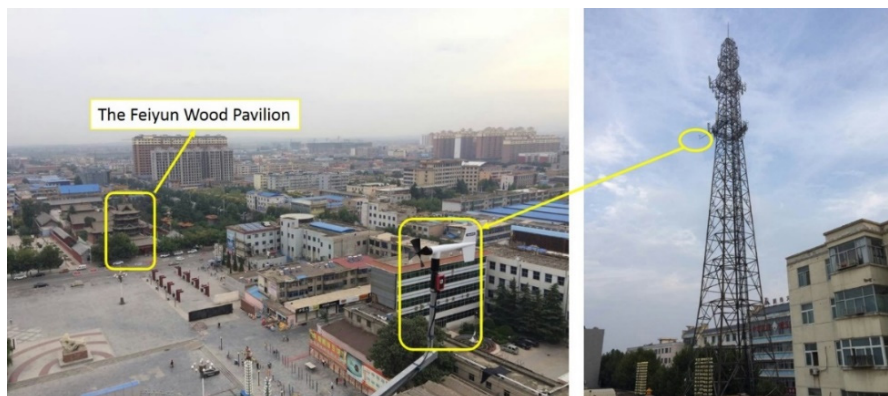
Fig. 7 Installation of anemometer
