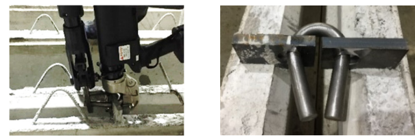
(a) Installation (b) Installed
