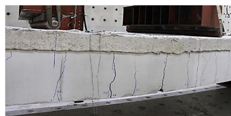
(c) Cracks of CM-550
