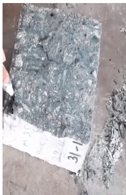
Fig. 9 Defining the crack place
