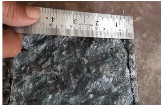
Fig. 12 The crack size 20 mm in concrete type 1 (steel 1% specimen)
