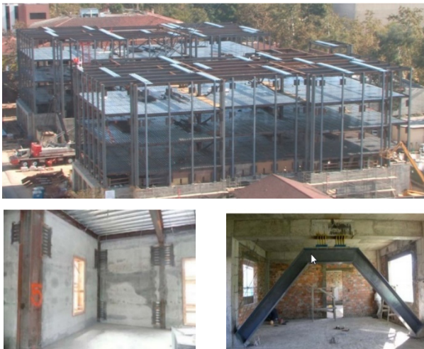
Fig. 2 The implementation of the butterfly-shaped fuses in USC School of Cinema (Luth et al. 2008)
