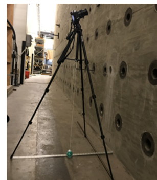
Fig. 4 A test large scale concrete structure including many cracks
