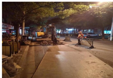
(a) Excavator breaking hammer
