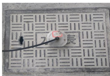
(c) The sensor placed on the manhole cover
