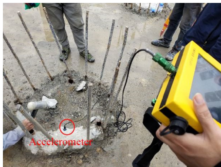
Fig. 25 The setup of the pile test
