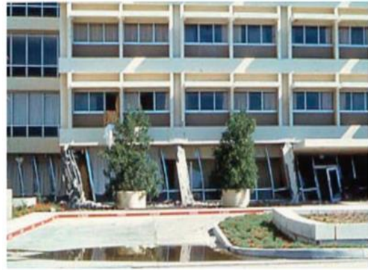
Failure of Olive View Hospital due to vertical geometric irregularity, 1971 San Fernando earthquake (FEMA 454 2006)
