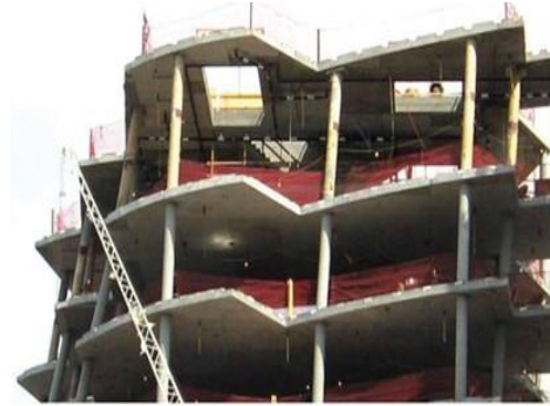
Building with excessive cut-outs (Portland Cement Association 2006)
