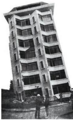
Failure of apartment building in Vina del Mar, Chile due to torsional irregularity, 1985 Mexican earthquake (Wood et al. 2002)
