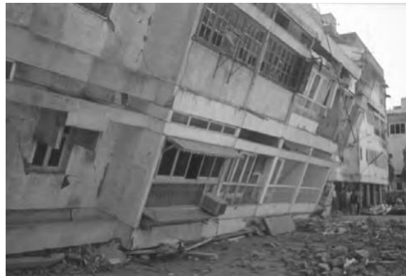
Collapse of ground floor of apartment due to soft storey, 2006 Bhuj earthquake (Agarwal and Shrikhande 2011)
