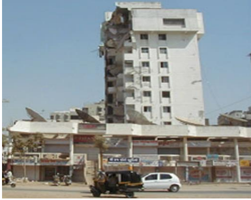
Collapse of half portion of Mansi complex due to presence of massive swimming pool at 10 th floor, 2006 Bhuj earthquake (Agarwal and Shrikhande 2011)
