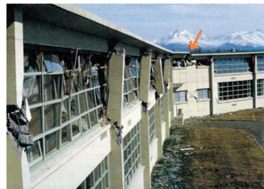
Concrete roof of a high school damaged due to stress concentration at re-entrant corner, 1964 Alaska earthquake (FEMA 454 2006)
