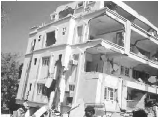
Damage of apartment due to floating columns, 2006 Bhuj earthquake (Agarwal and Shrikhande 2011)
