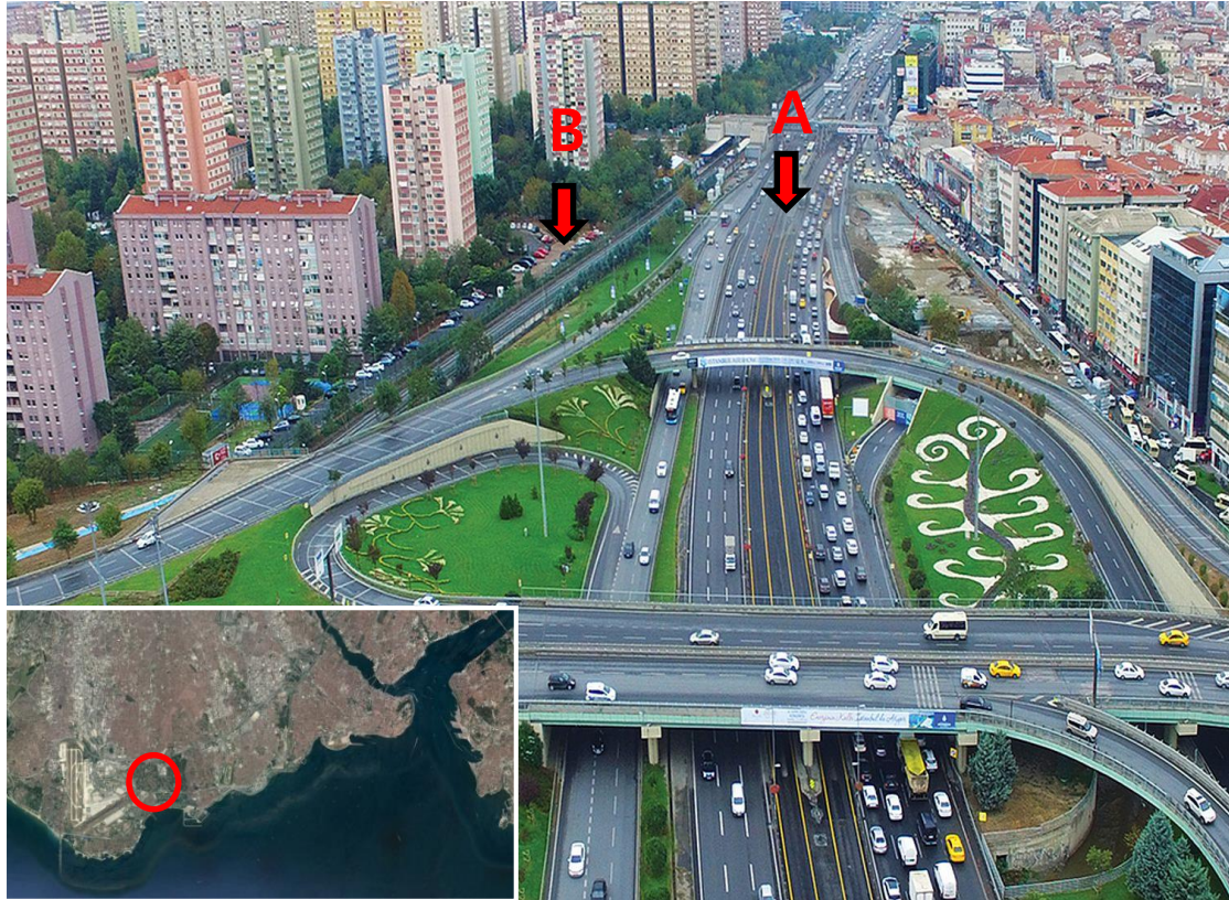
Fig. 1 An aerial photograph of the highway, red arrows show the location of the measurement stations A and B (inlet) The location of the Atakoy district
